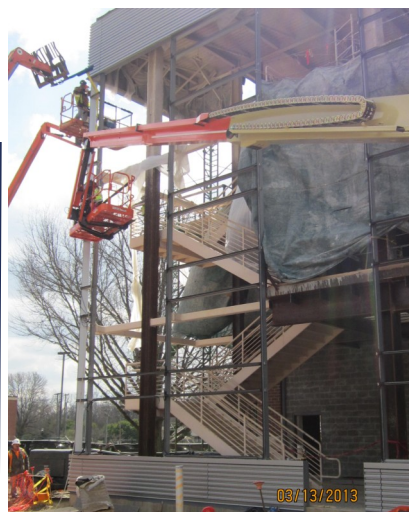
Above; Workers install the glass curtain wall system at the stairwell on the east end of Area D. This curtain wall system will stretch around almost all of the building on the courtyard side of the building.
