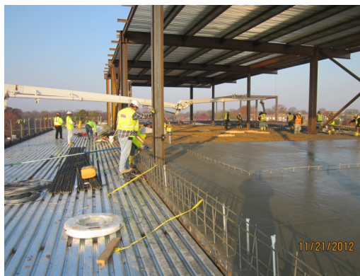
Above: Concrete workers place and finish the penthouse slab, which required 133 cubic yards to be pumped up 4 stories
