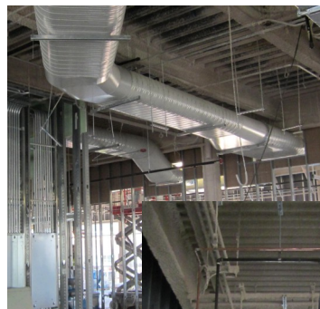
Left; Ductwork and plumbing are making their way through Area D 2nd and 3rd floors. This will soon be an extremely intricate maze of pipes, ducts, and conduit in order to feed the building.
