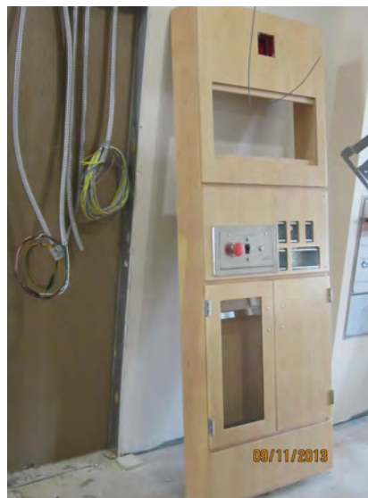
Above: Ceiling grid starting to be installed in the Area D 2nd Floor Labs.. Below: A Safety Station is set for installation. These will include emergency shut-offs, projector and shade, controls, among others.
