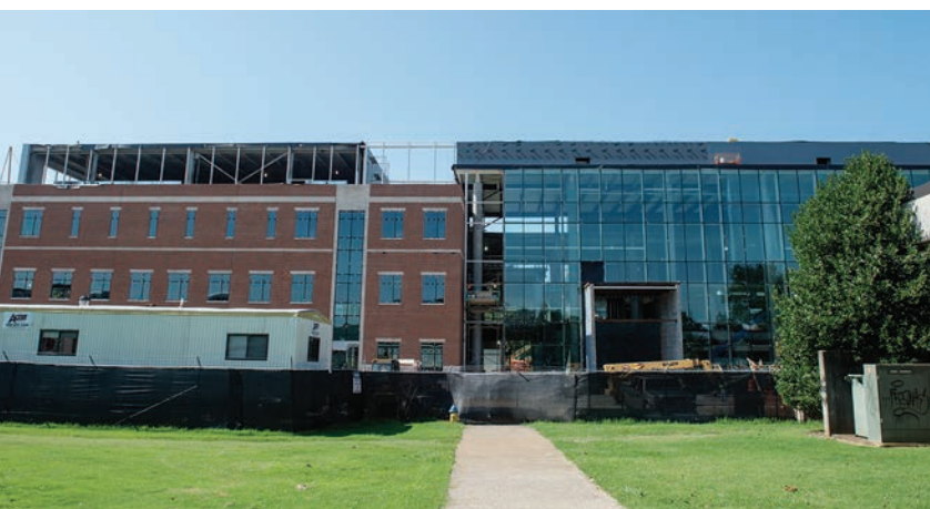
Construction of the new science building, due to be completed in 2015.
