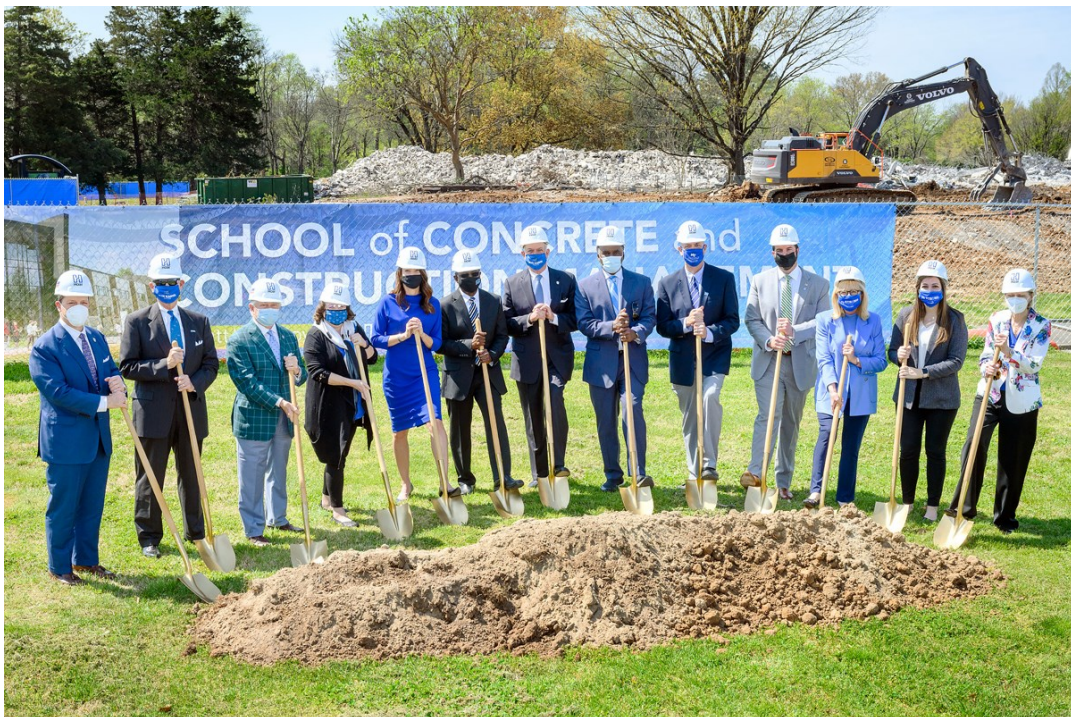
MTSU officials celebrated the groundbreaking ceremony for the 54,000-square-foot, $40.1 million School of Concrete and Construction Management Building on the southeast side of campus Tuesday, April 6. Ceremonial shoveling of dirt participants included, from left, Pete DeLay, trustee; Tom Boyd, trustee; J.B. Baker, trustee; Mary Martin, faculty trustee; Heather Brown, professor of concrete industry management; MTSU President Sidney A. McPhee; Stephen Smith, Board of Trustees chairman; Darrell Freeman, trustee vice chairman; Kelly Strong, director, MTSU School of Concrete and Construction Management; Daniel Bugbee, CIM (Concrete Industry Management) Patrons president; Pam Wright, trustee; Delanie McDonald, student trustee; and Christine Karbowski Vanek, trustee. (MTSU photo by J. Intintoli)
